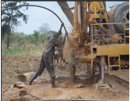
Borehole at St Mary's Primary School
