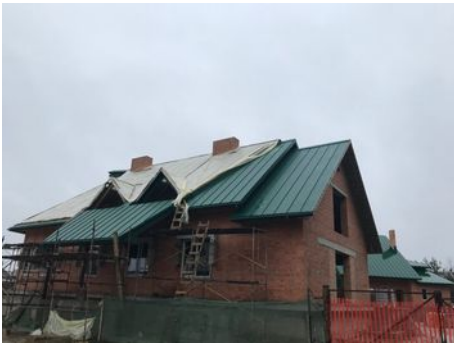
The new building takes shape
